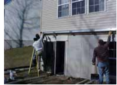
Ledger support is installed
