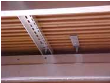
Deck is fastened from underneath
