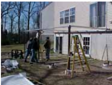
Sub-frame is erected
