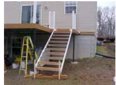
Prefabricated stairs installs in minutes
