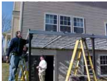
Stringer frame is installed
