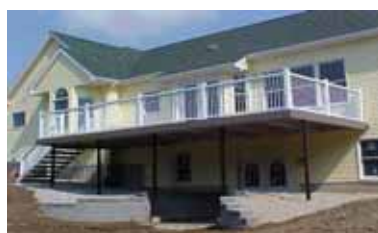
Finished deck has clean low profile look
