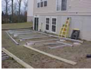
Deck is laid out
